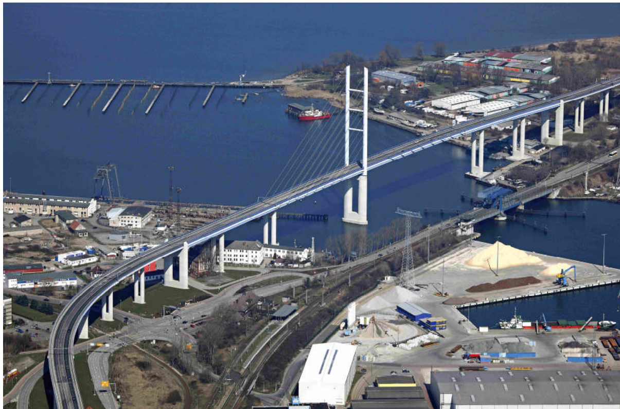
Figure 1: Cable-stayed Ziegelgraben bridge
