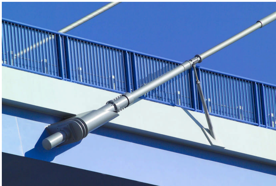
Figure 8: Cable anchorage with cantilevered hydraulic damper
